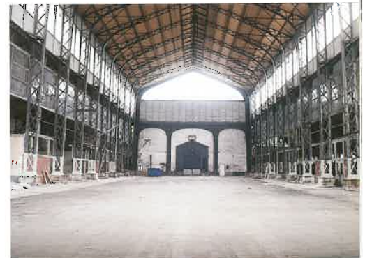
Figure 4 Vaisseau principal du hangar Y. © Brice Desrez/ Drac Ile-de-France.
